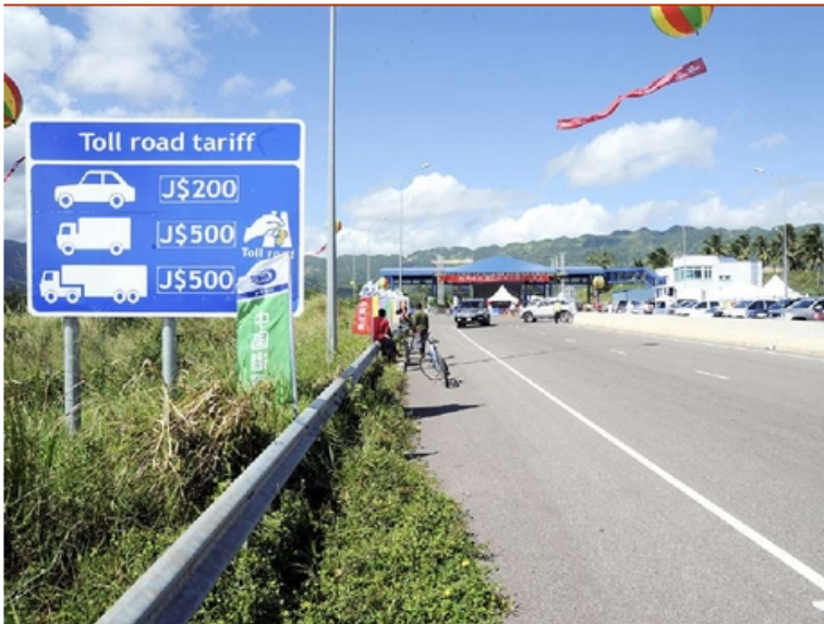
This section of the north-south link of Highway 2000 will enable motorists to bypass Mount Rosser. It connects Treadways, St Catherine, to Moneague, St Ann. - Norman Grindley/Chief Photographer
